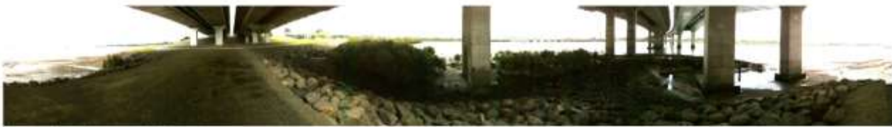
View under Motorway Bridge
