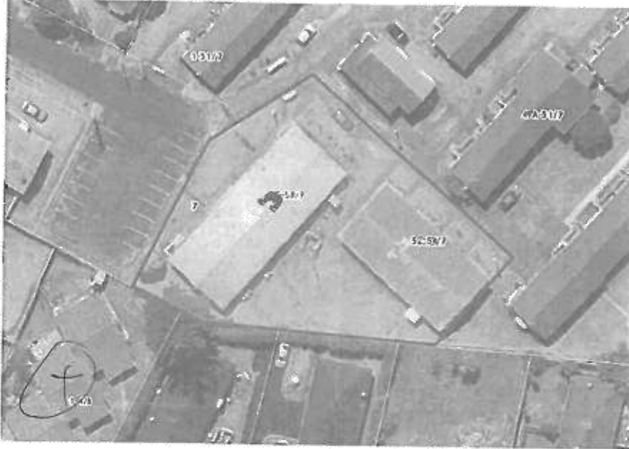
Images of Units 56 and 57, 7 Rowlands Avenue, Mt Wellington
