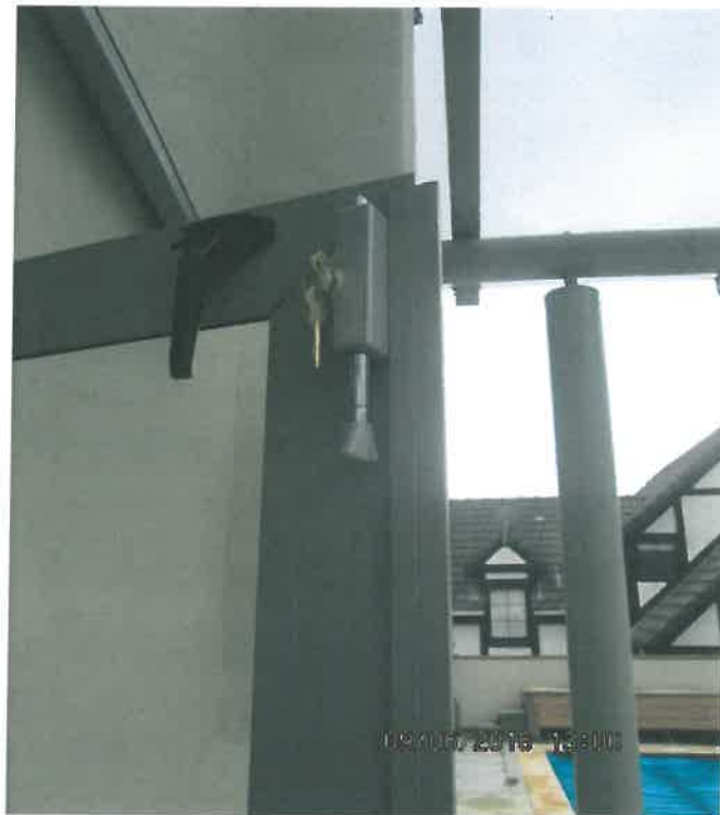
Lockable top bolt fitted to other door
