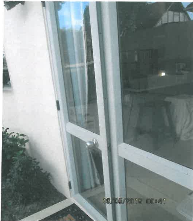
Door opening into pool area
