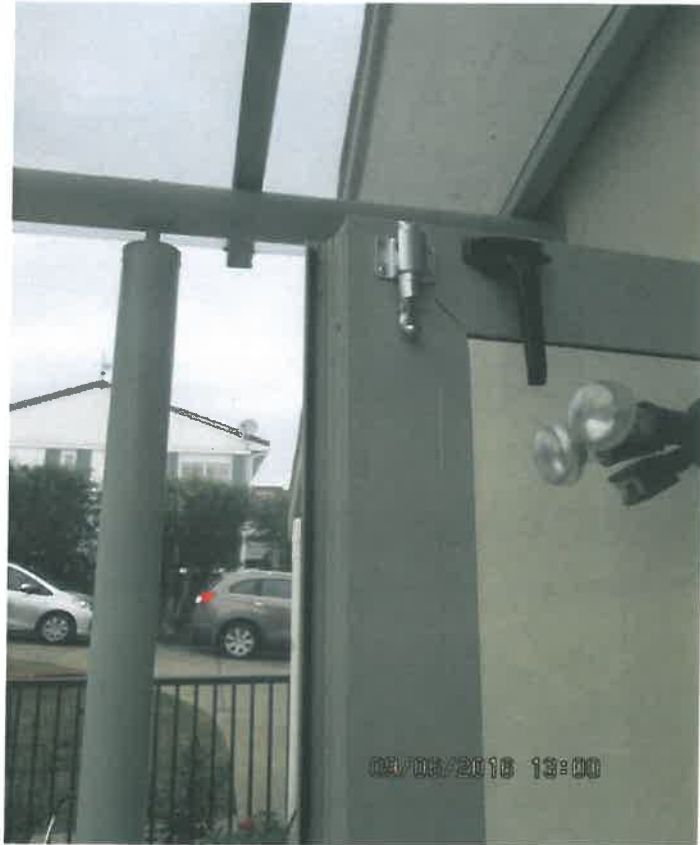
Self-latch device fitted higher than 1.5m
