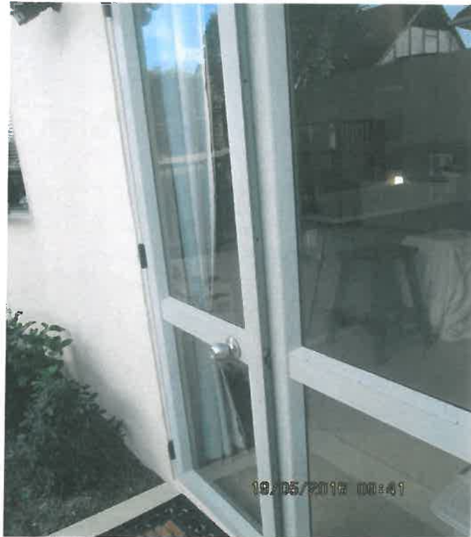
Door opening into pool area
