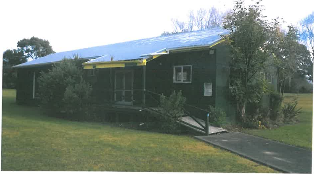
Attachment G image of existing scout den on Riverpark Reserve, Henderson for potential relocation to Blomfield Reserve
