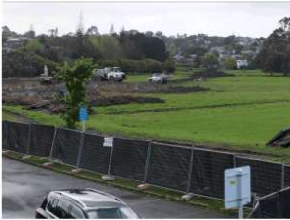
Figure 6 Sunnynook park project
