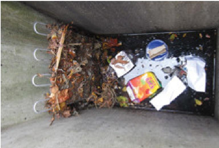
**Image 1 showing an installed tetra trap trapping pollutants from entering waterways**
