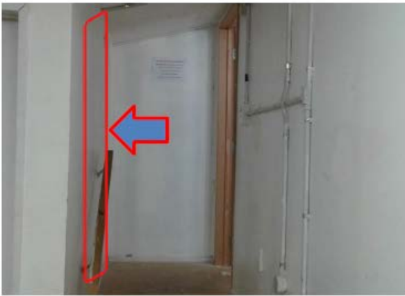
New fire exit door on top of the landing
