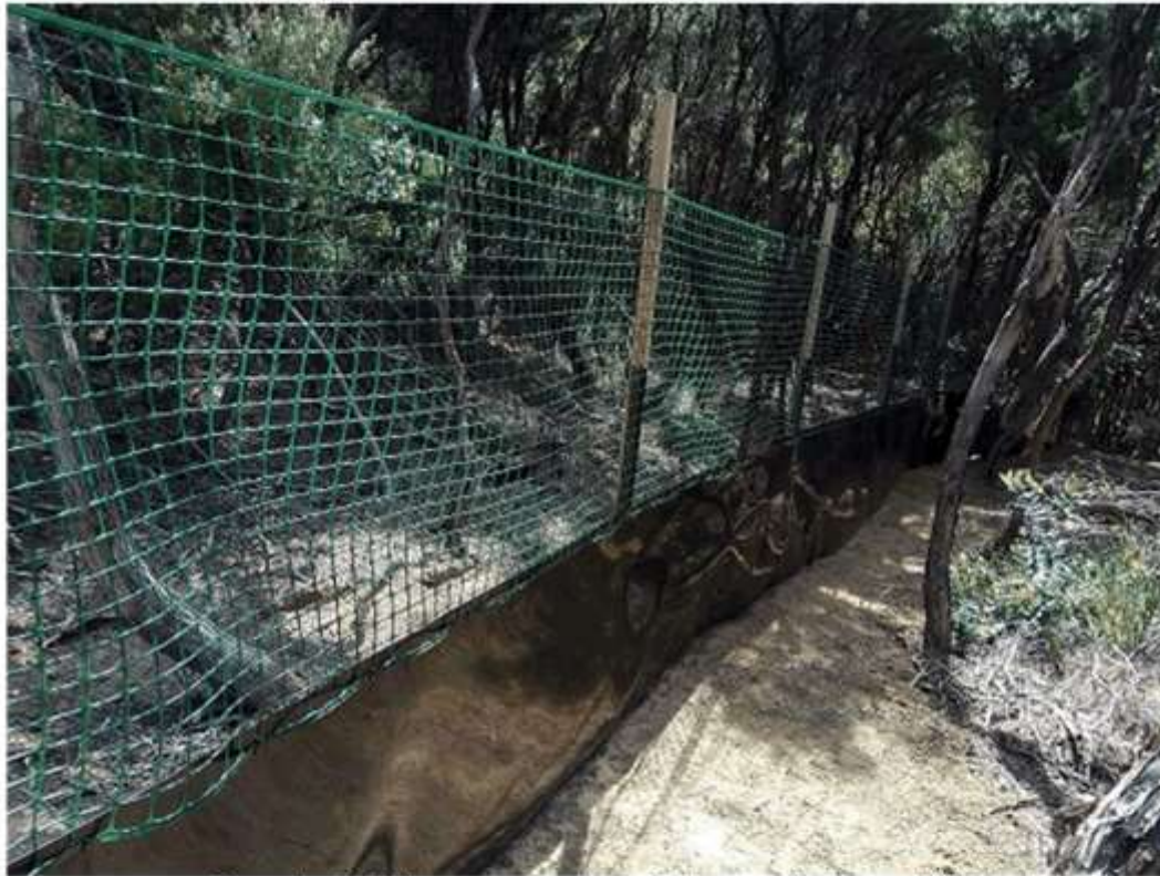
Example of chicken coop fencing: chicken mesh above skink fencing
