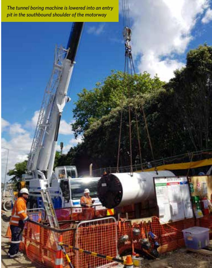
The tunnel boring machine is lowered into an entry pit in the southbound shoulder of the motorway
