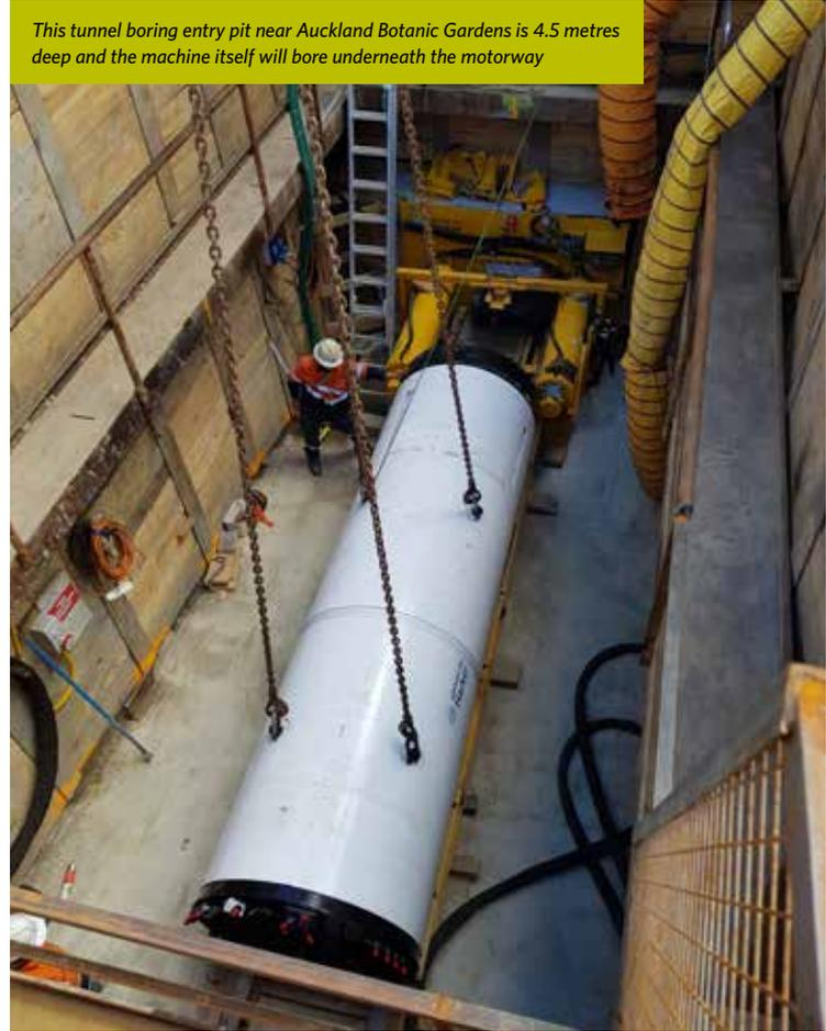
This tunnel boring entry pit near Auckland Botanic Gardens is 4.5 metres deep and the machine itself will bore underneath the motorway
