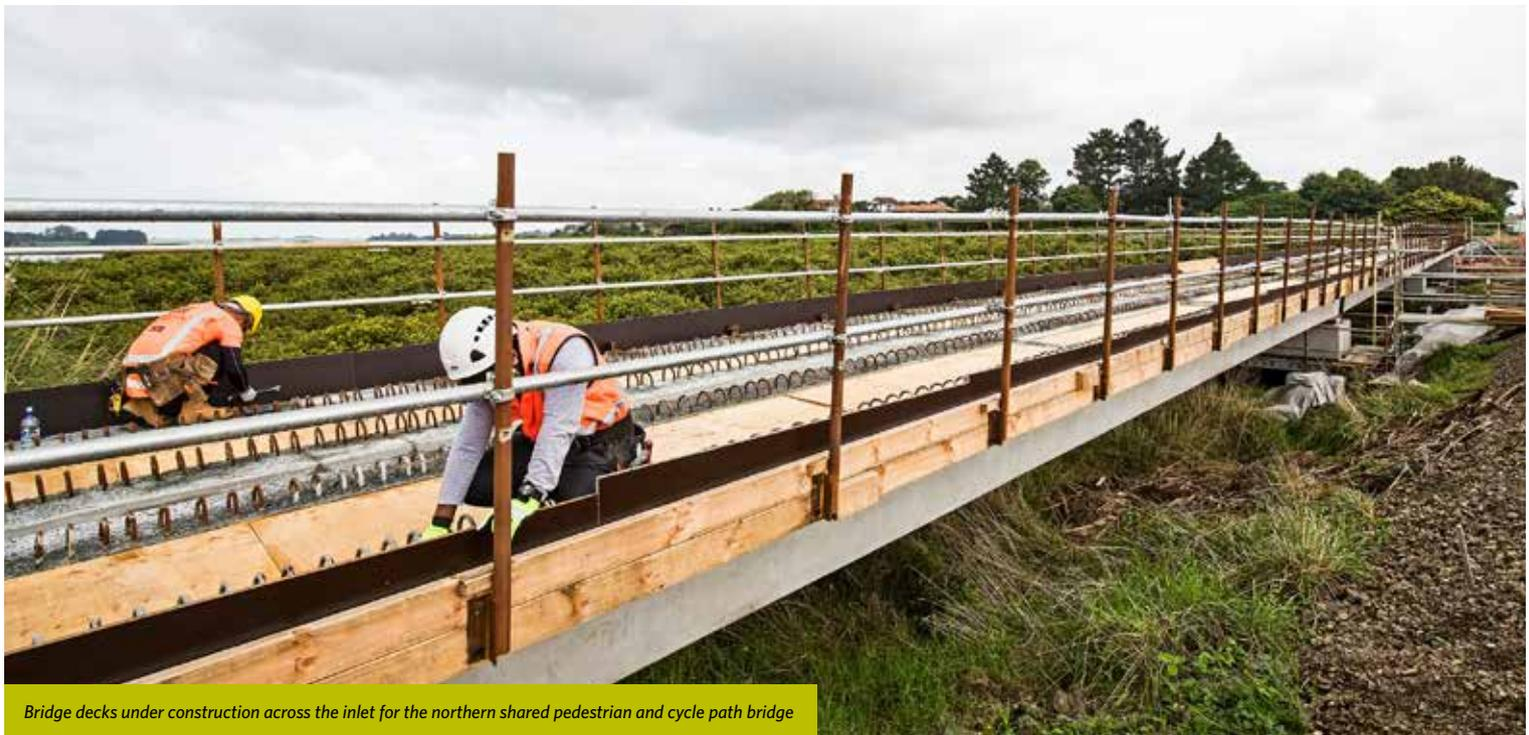
Bridge decks under construction across the inlet for the northern shared pedestrian and cycle path bridge
