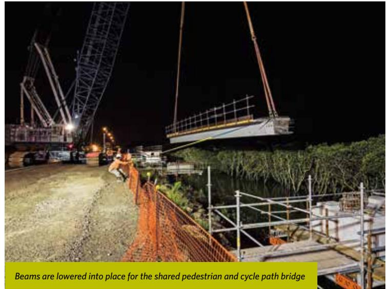
Beams are lowered into place for the shared pedestrian and cycle path bridge
