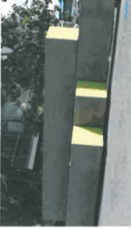
Timber stack seat - North Wharf
