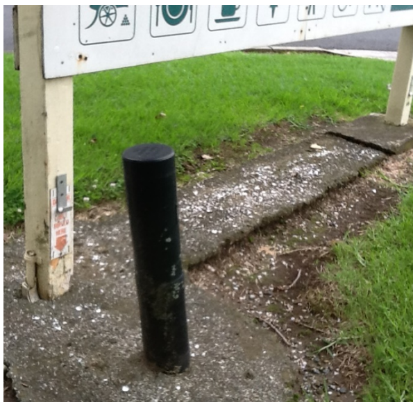
Figure 3. The signs will be installed with concrete mowing strips.
