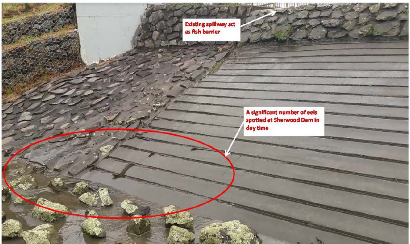
Photo 1: Fish Barrier at Spillway and Sherwood Dam
