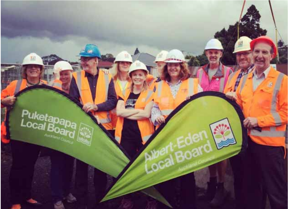
Owairaka Footbridge installation – With Puketapapa Local Board
