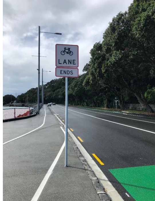
Poorly placed sign in Tamaki Drive
