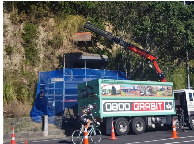
Debris removal searchlight no. 2
