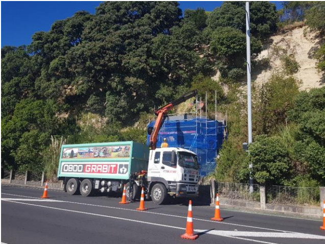
Debris removal searchlight no. 1
