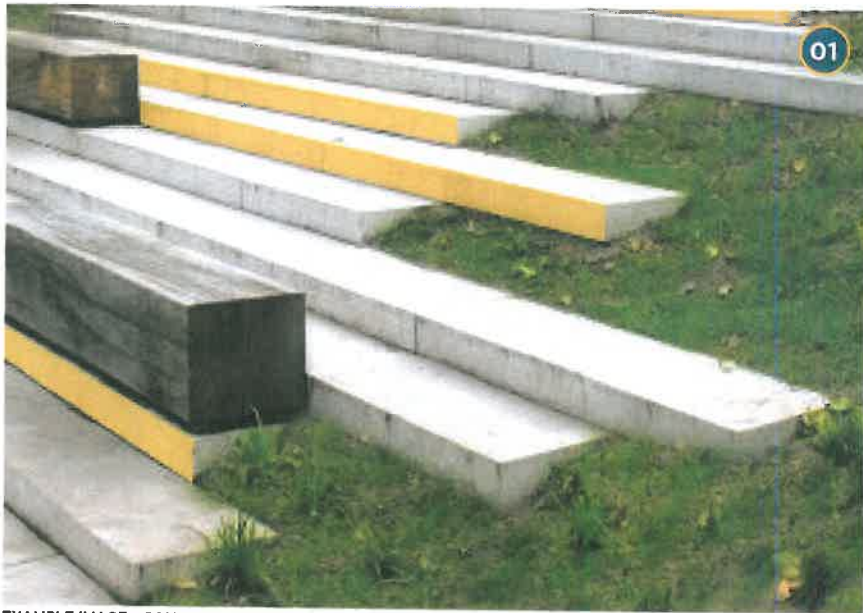
EXAMPLE IMAGE - CONCRETE STEPS LEADING DOWN FROM EXISTING SWING. PAINTED FACES.
