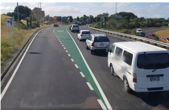
Figure 3: Short section of bus only lane / queue jump in advance of the Esmonde Road off ramp traffic lights enabling buses a free run to the front of the queue where they turn right towards Akoranga Bus Station.
