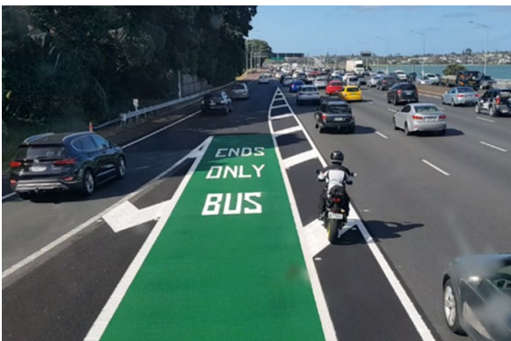
Figure 2: The bus only lane has been extended further into the Onewa Road on ramp lane making the merge into general traffic much easier
