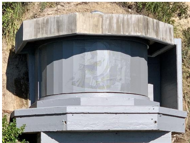
Emplacement 2 - after restoration with artwork showing an image of a soldier operating one of the searchlights
