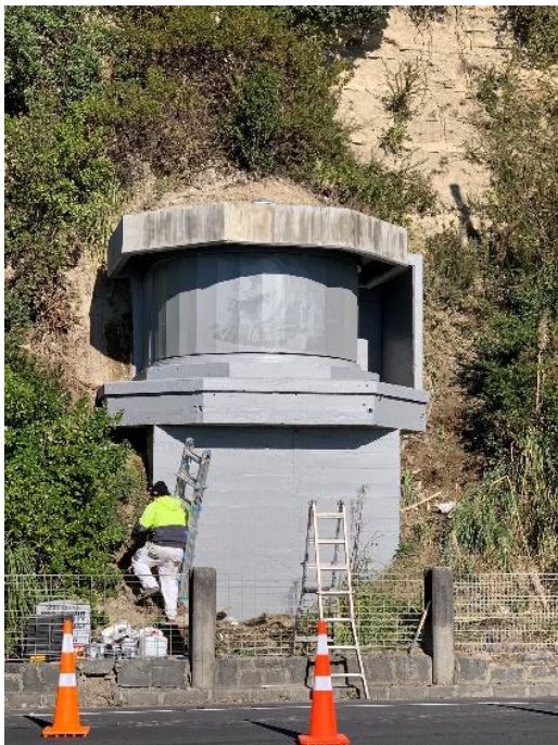
Emplacement 2 - during restoration
