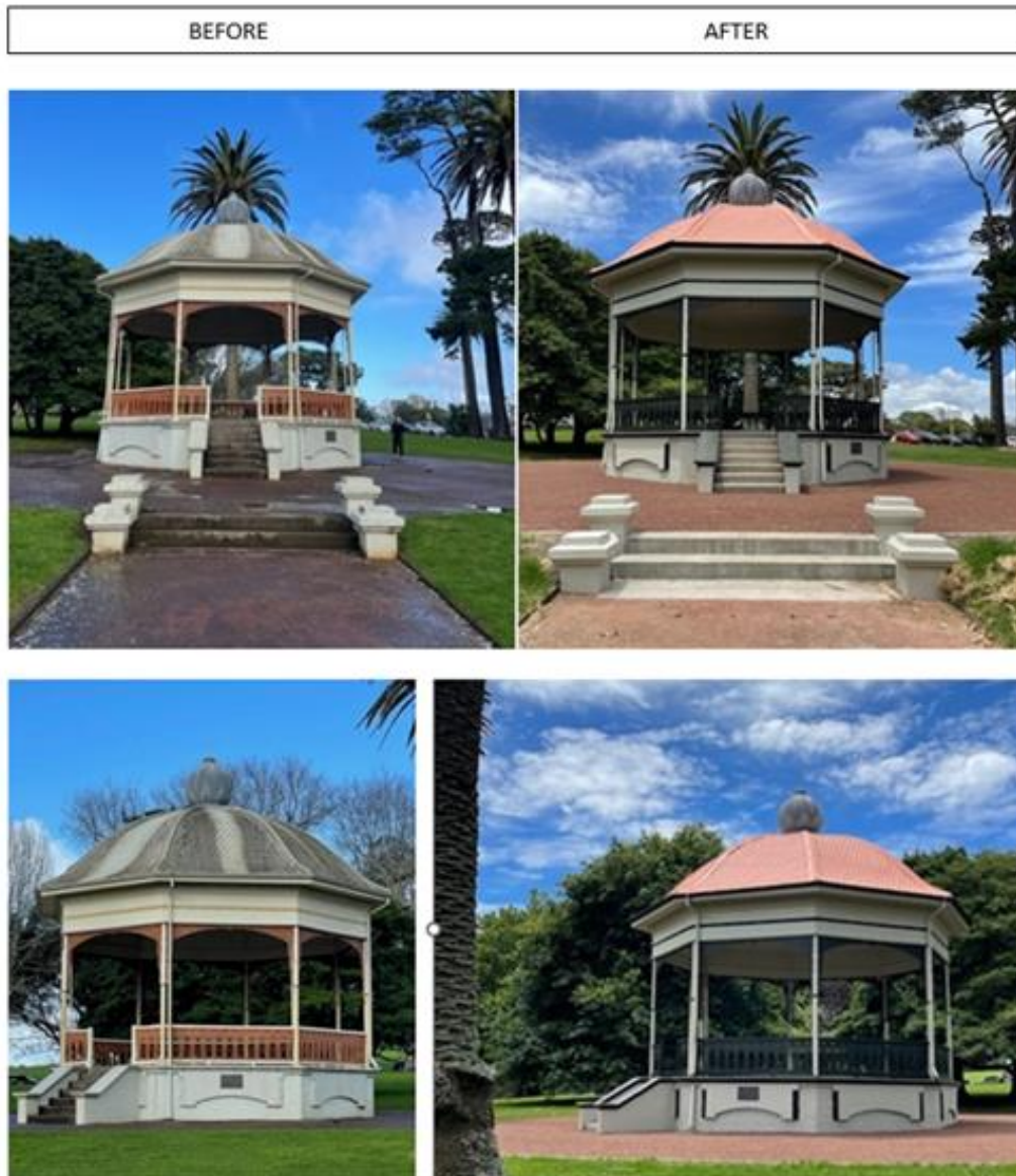
Before and after photographs of the band rotunda upgrade.
