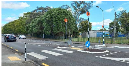
Warning Tactile Pavers:
