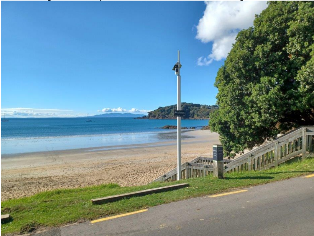
Figure 4: Coastal monitoring camera installed at Oneroa
