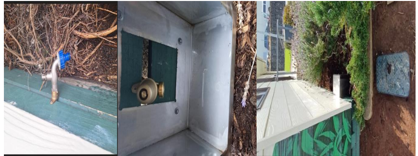
Drury Library. To mitigate the rough sleepers in this area. We installed a lock box around the outside garden tap.
