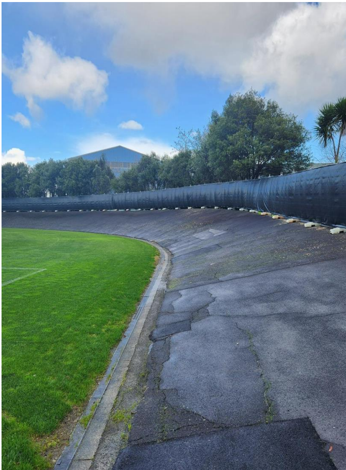
Figure 2. Photo demonstrates the poor condition of the velodrome's surface (Source: Visitor Solutions).
