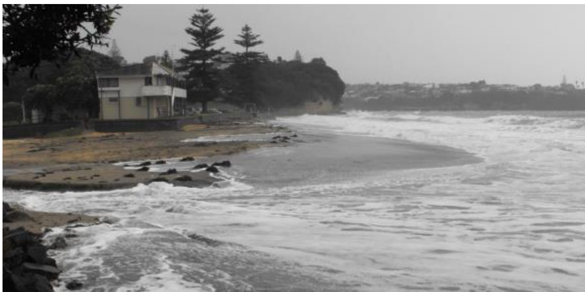
Figure 2 – the Mairangi Bay Surf Lifesaving Club building during a 2016 storm event (source: Matt McNeil, Auckland Council)
