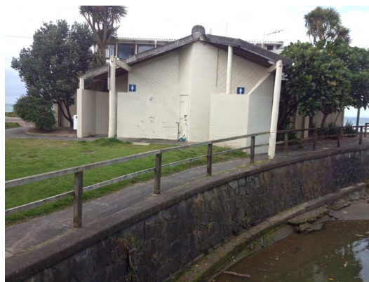
Public toilets adjacent to the surf club
