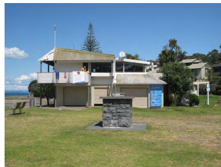
The public barbeque is located 20 metres from the surf club and public toilets
