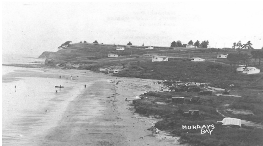
Looking south from Montrose Terrace over the beach settlement of Mairangi Bay Beach Reserve (formerly known as Little Murrays Bay) in the 1920s. Whitby Crescent provides access to baches on the hill in the background. (Auckland Libraries – North Auckland Research Centre ID# 233)
