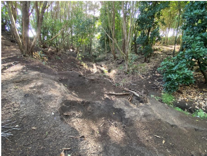
Extensive areas of trees destroyed by earthworks for construction of BMX track network. No regeneration. All photos below are from the Forfar Gully.
