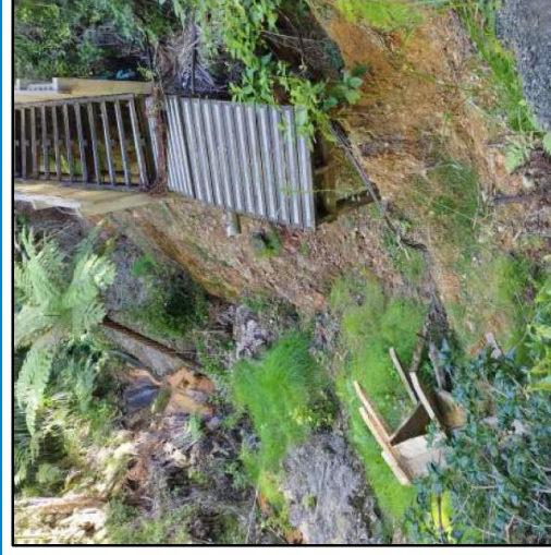
(Right Photo: shows the exposed pipe and the undermined pathway. Left Photo: shows the extent of the scouring downslope of a bridge. Date Taken: 15/01/2024)
